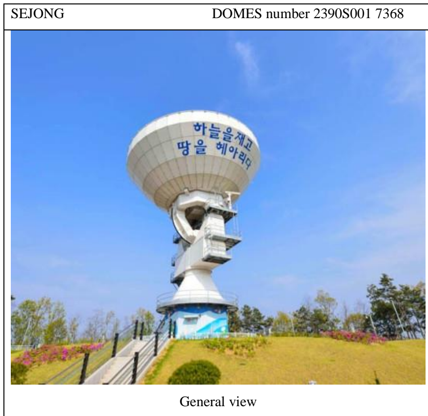
Figure 3. VLBI station installed at Sejong Space Geodetic Observatory
