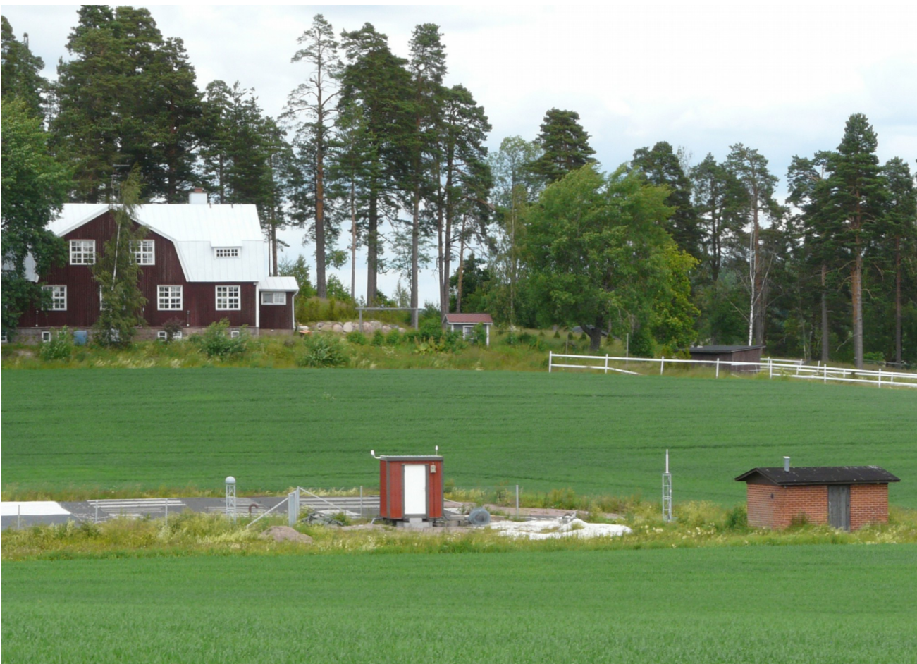
From left to right : GNSS antenna, shelter, DORIS antenna.
